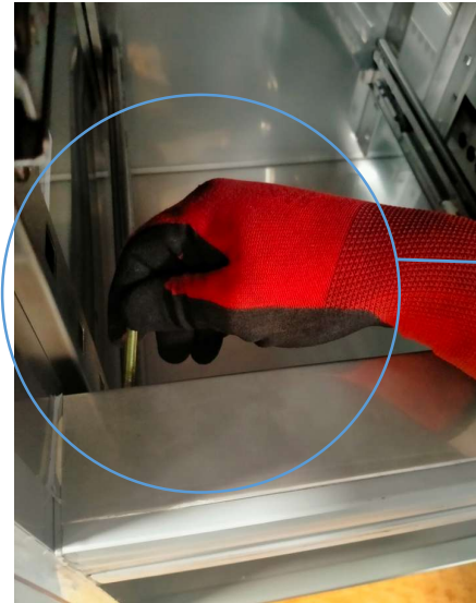
Photo 12: Spacer fixation.
