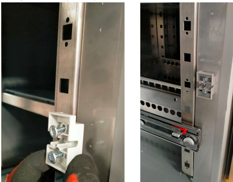
Photo 8: Installation of spacer supports.
