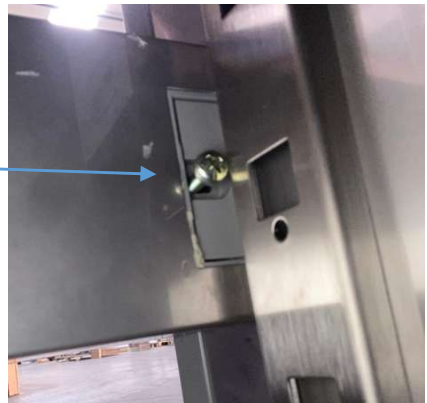
Photo 12: Spacer fixation.
