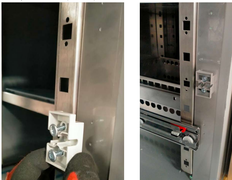
Photo 8: Installation of spacer supports.
